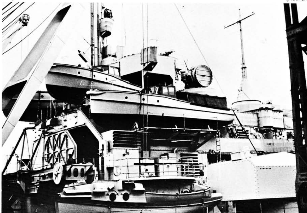
The after-superstructure, showing the sliding hangar door, the boat stowage and the signalling projector on the mast. Early 1940 (Author)
